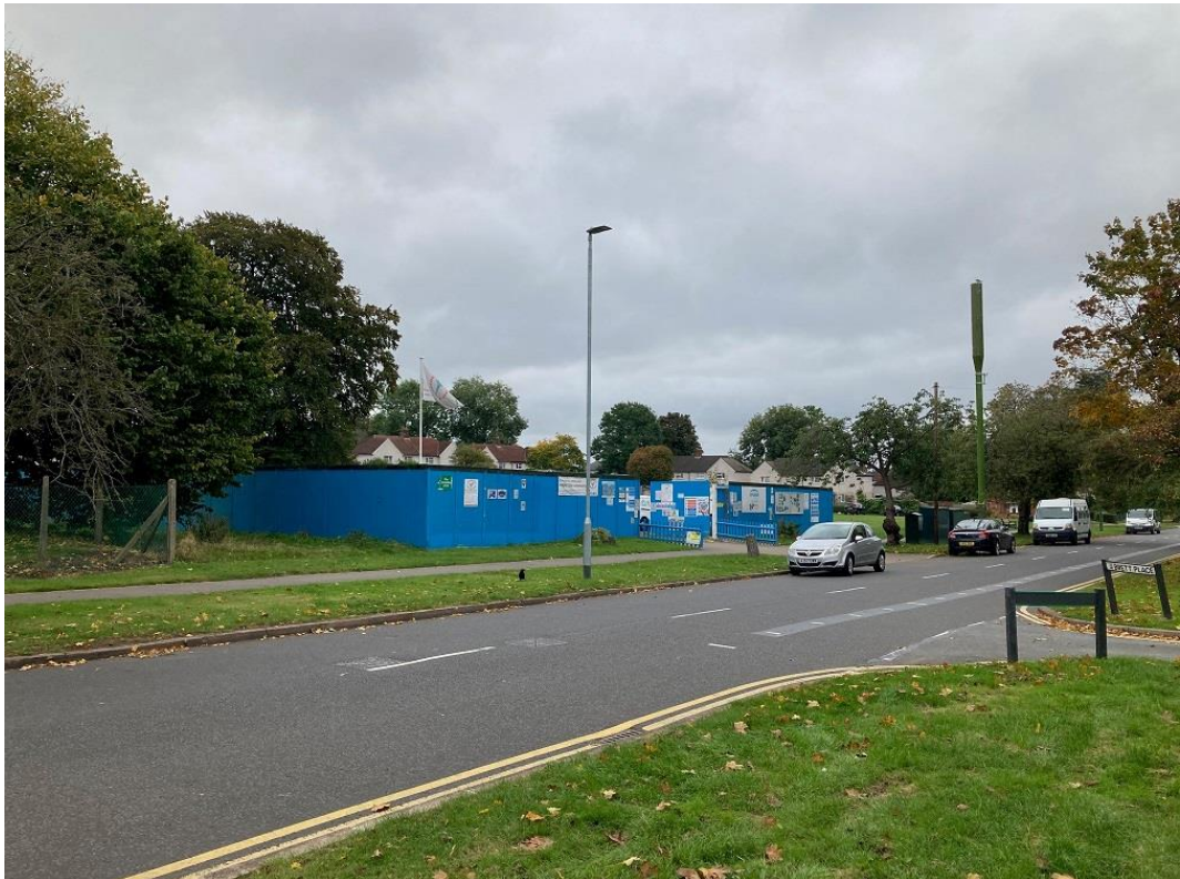
View of Compound looking East
